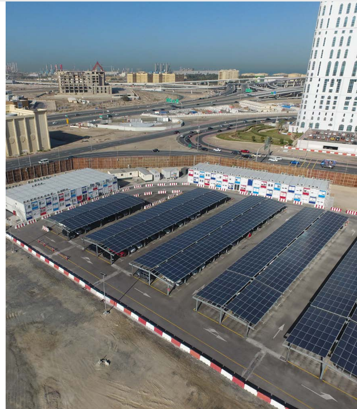
BEsim, Uptown Tower, Dubai (UAE) BEsim – BESIX site installation management Standardize and improve BESIX's site installation: encouraging re-use of offices and site setups. Results: lower the overall cost of site installation, improve comfort of employees, lower carbon footprint, reuse of equipment and renewable energy.
