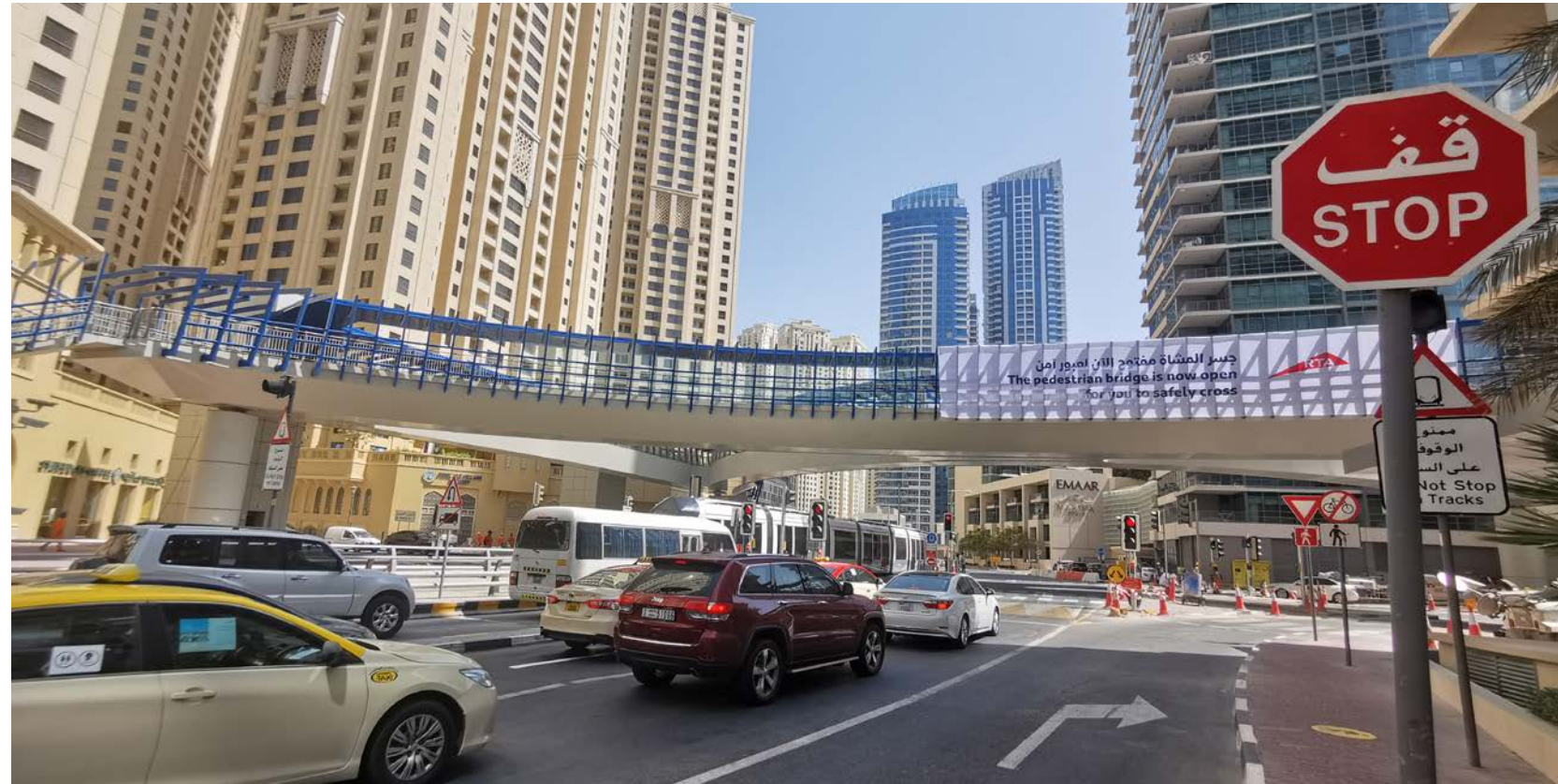
Dubai pedestrian bridge (UAE) – A four-way footbridge (75 m length) that allows +8,000 pedestrians to safely cross one of the busiest junctions in Dubai. This project is to be part of the Dubai Roads and Transport Authority's plans to rank among the world's safest cities in traffic safety by 2021.
