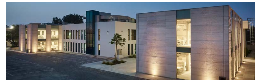
BESIX 3D printed the largest 3D printed concrete façade in the world for the new Dubai headquarters of BESIX in 2020. Results: use less concrete and carbon footprint reduction with more complex shape opportunities.
